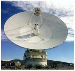
One of the 70-m diameter Deep Space Network antennas that communicate with faraway spacecraft. As Earth turns, an antenna at one of three DSN locations around Earth acquires the spacecraft's signal, as the downlink is lost by the antenna rotating out of view.
